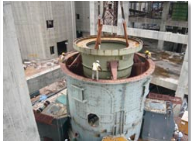
Figure 9: Lifting and lowering of grinding table
