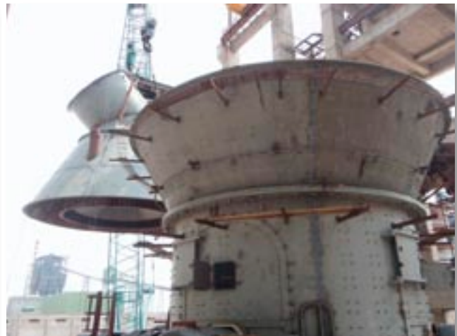
Figure 11: Erection of classifier on mill housing
