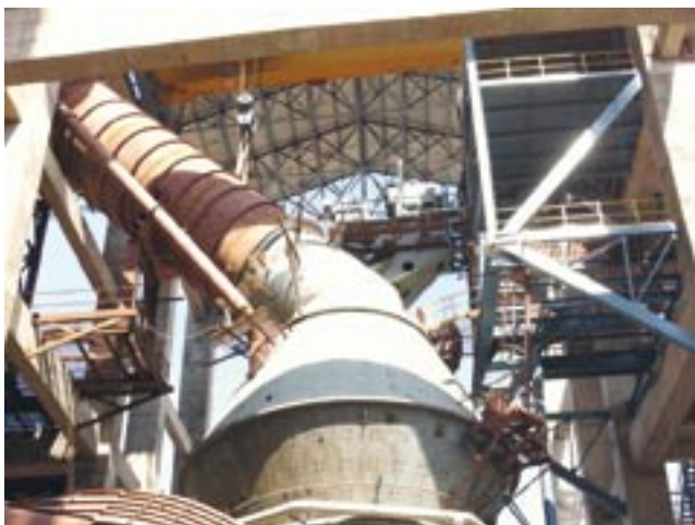
Figure 12: Feeding arrangement for dry fly ash
