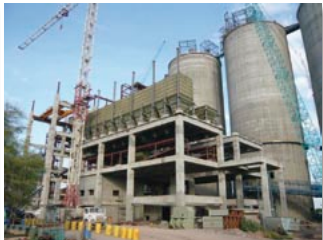
Figure 13: Erection of bag filter
