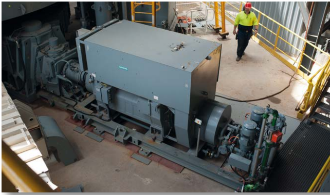
Figure 10: Motor accessibility with the MultiDrive® drive system
