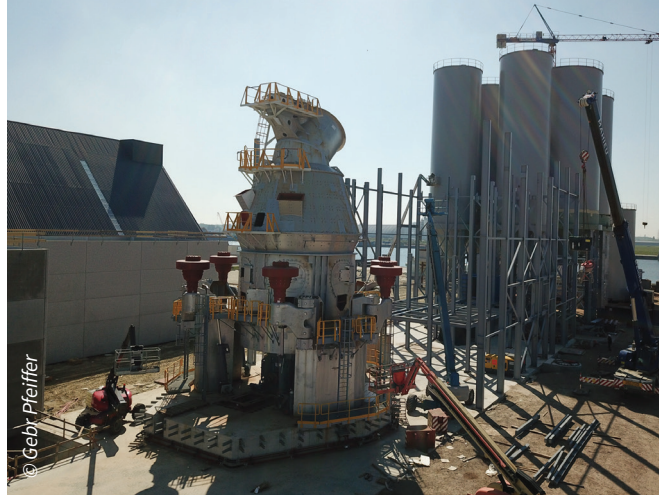
Figure 3: the MVR 5300 C-6 and silos during erection
