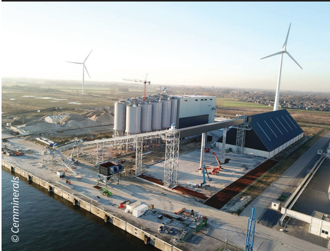
Figure 2: view of the grinding terminal in western Europe under construction
