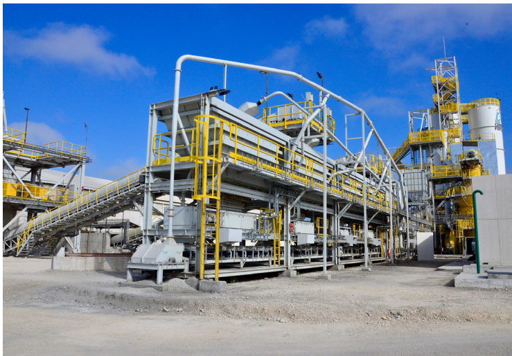
Figure 6. Crusher and feed hoppers.
