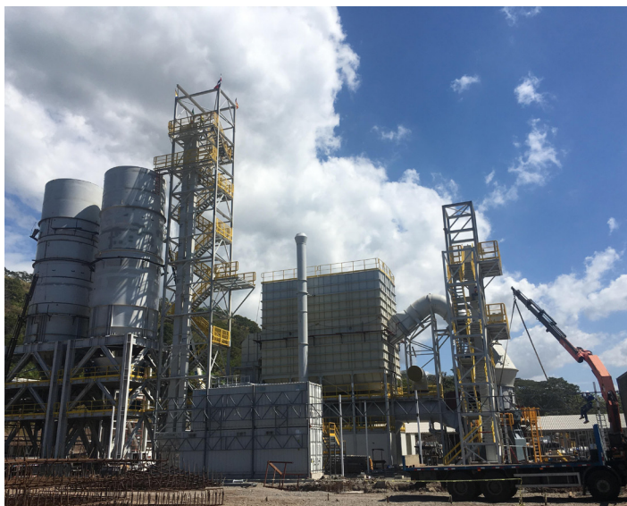
Figure 2. R2G 2500 C-4 under construction in Costa Rica.
