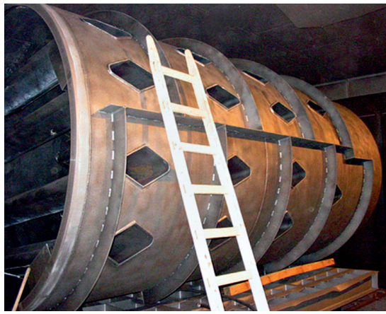
4 The kettle with its hot gas pipes
