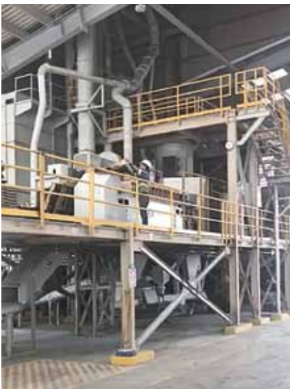
The packing area is housed in a covered cement storage building
