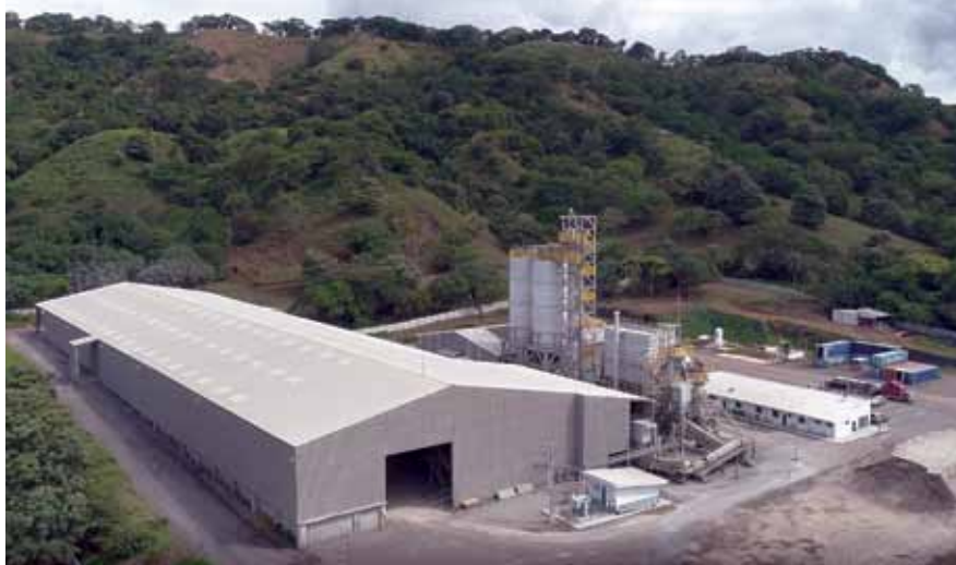
Clinker storage and mill feeding area of Gebr Pfeiffer’s ready2grind system at Elementia’s Salinas Esparza plant, Costa Rica
