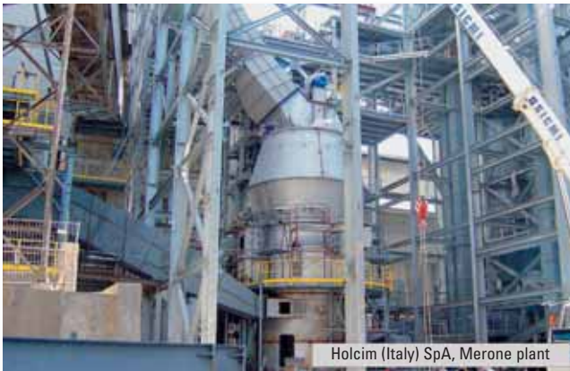
Figure 3: Assembled mill in the steel structure
